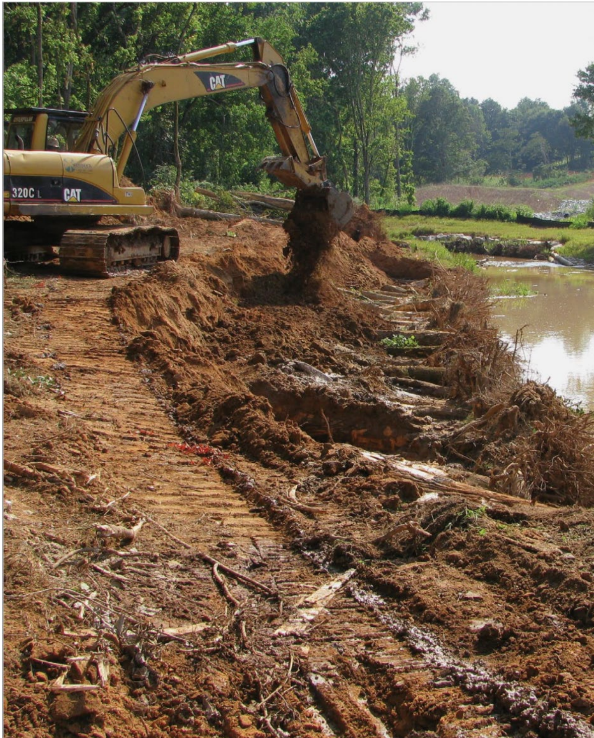
Figure 7. Streambank stabilization via rootwad. Harris County Flood Control District – Streambank Stabilization Handbook
